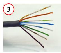
Position Wires into Correct Configuration (TIA 586-B Shown)
